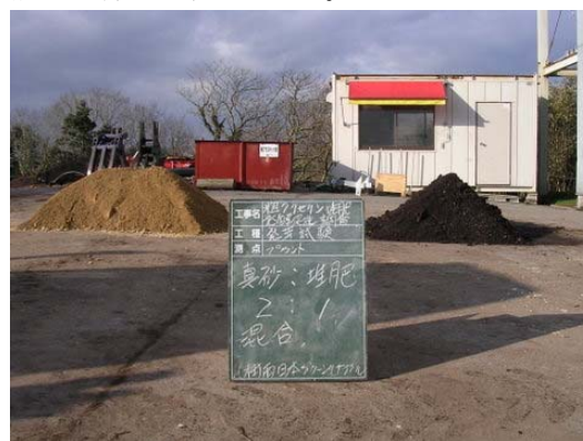
Photo 5. The soil and compost before mixing.
