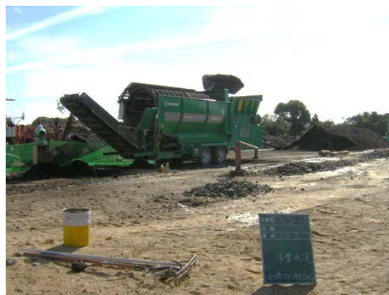
Photo 4. The work scenery of the riddling by use of sieve machine.
