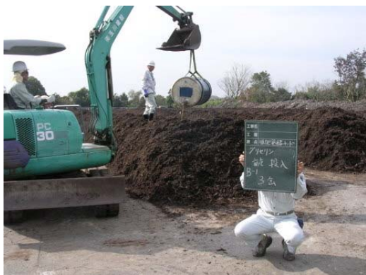
Photo 2. The work scenery of adding glycerol waste liquid to test fields.
